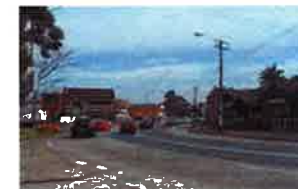
1 The wide, busy traffic thoroughfare of Victoria Road
