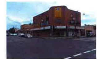
2 Corner Victoria and Sydenham Roads
